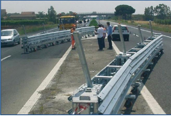
Each module is formed from a triple wave steel beam strip with a further steel longitudinal running beam that is designed to the wheels of any impacting vehicle. The sides of the module are joined by strong steel supports which include the mounting supports for the hinges and the removable frame posts.
