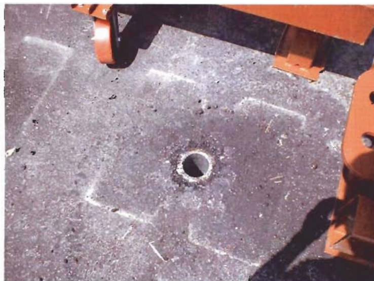
Figure 2 – Inserted sleeve
