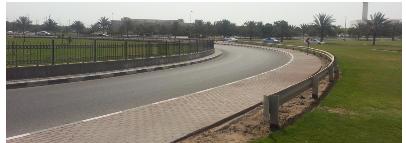
Full height hazard with inadequate anchorage for the guardrail system to perform.
