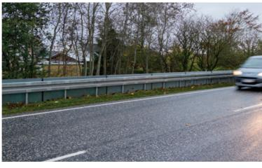
80 % of all traffic noise on roads comes from the interaction of the asphalt and the wheels of passing vehicles. With a sound source that low, there is no need for a massive wall to block the noise, if a screen can be brought close enough to the traffic. The solution is the noise absorbing safety barrier EasyRail® NA.
